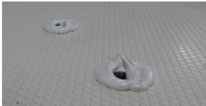
Apply a bead of sealant in between the holes and over the area of the platform which will be in contact with the extension plate (20).
